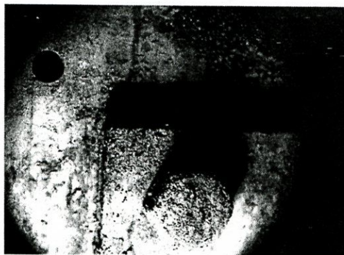
Fig. 8. The image of the good state of core painted surface (the base flange and the bolt) after 47 years of water action. The hole in the left upper side was drilled in the core plate steel and the concrete was found inside.
